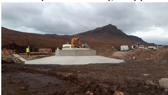
wind very soon: the track to the site is complete (for use by walkers, crofters, anyone after the turbine is up) the crane pad is finished and the underground cable is buried ready for plugging in. The foundations and base build are well underway in readiness for the turbine crossing the briny from Denmark (where it was built) to its new home in Achavraie. Prize for the best name suggested but NOT Windy MacWindface, please!
